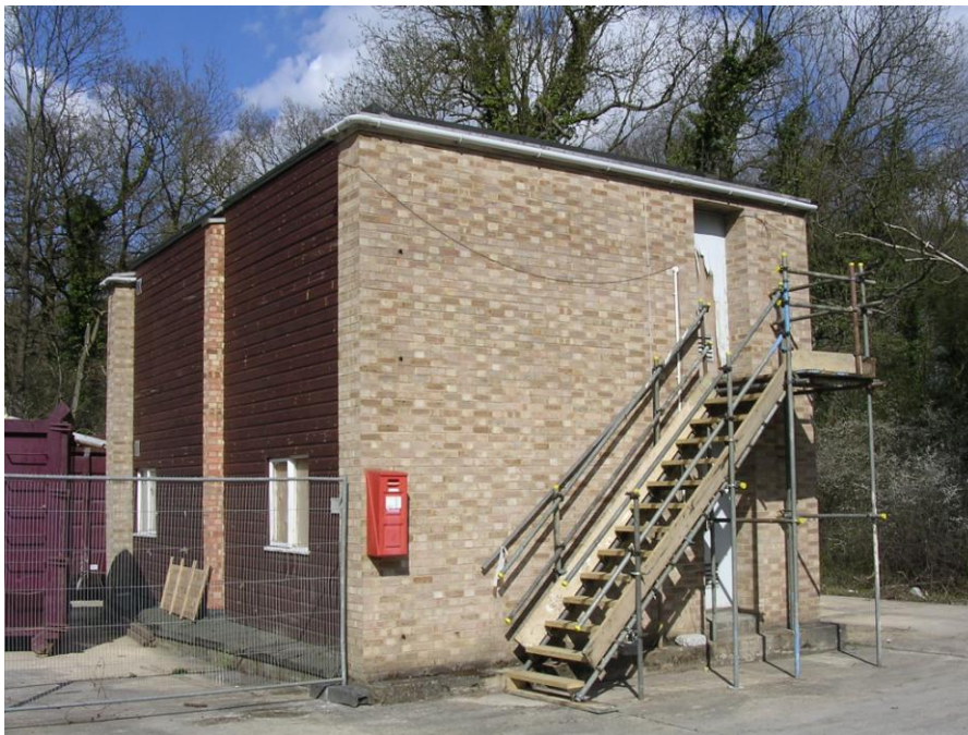
Photograph 1: Building 68, at BRE, Watford
